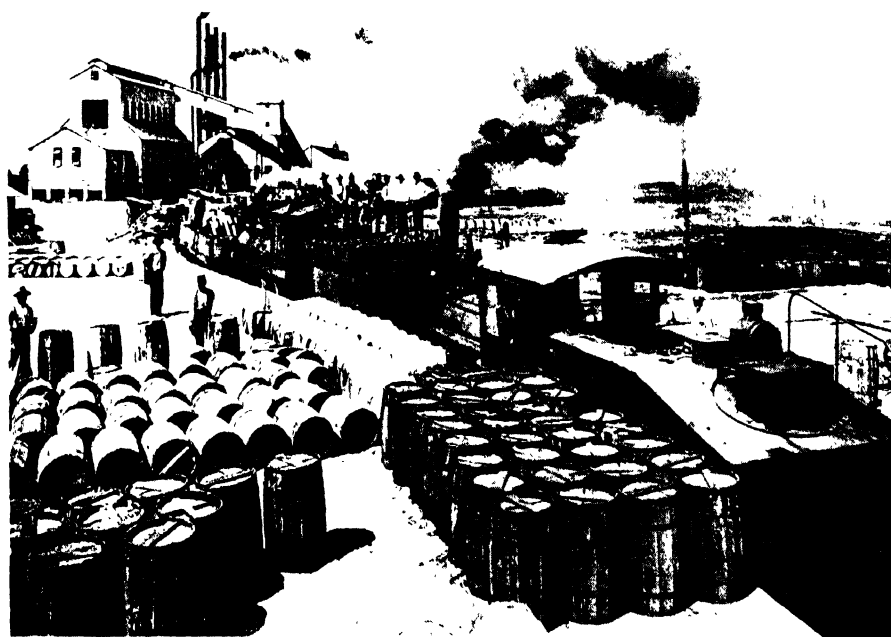
Pensacola Plant of Newport Industries, Inc.
